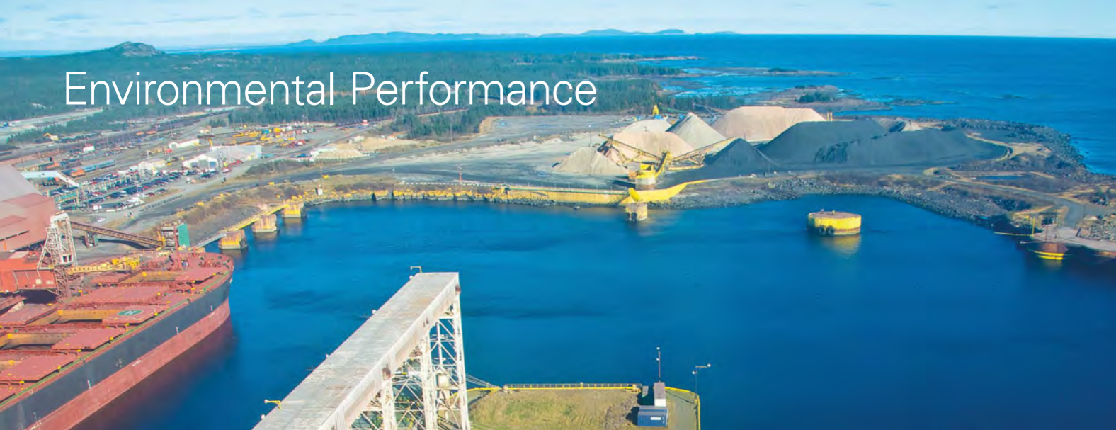
Our terminal in Port Cartier, Québec, Canada
